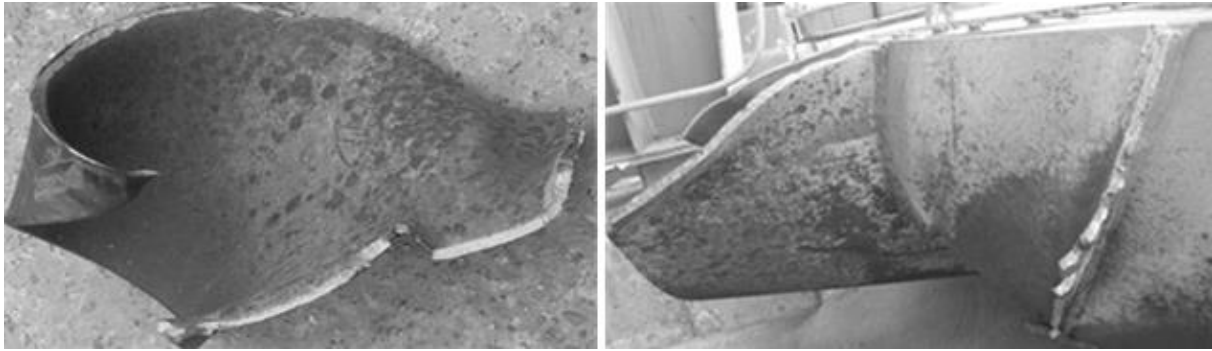
Figure 4. Example of fracture failure (left) and an example of breaking the blades from the root (right side).
